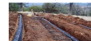
Layout pipelines and marking inverted levels (P4)
